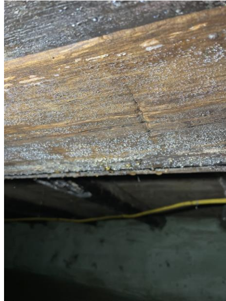
Surface moisture is collecting on the timbers and surfaces of the ceiling in the basement. This will certainly attract fungi, which will break down the heartwood and allow insect infestation if not remedied ASAP. There is no air circulation or movement due to the spray in foam. Even the windows were covered in spray-foam! This is a disaster for a timber-framed building.
